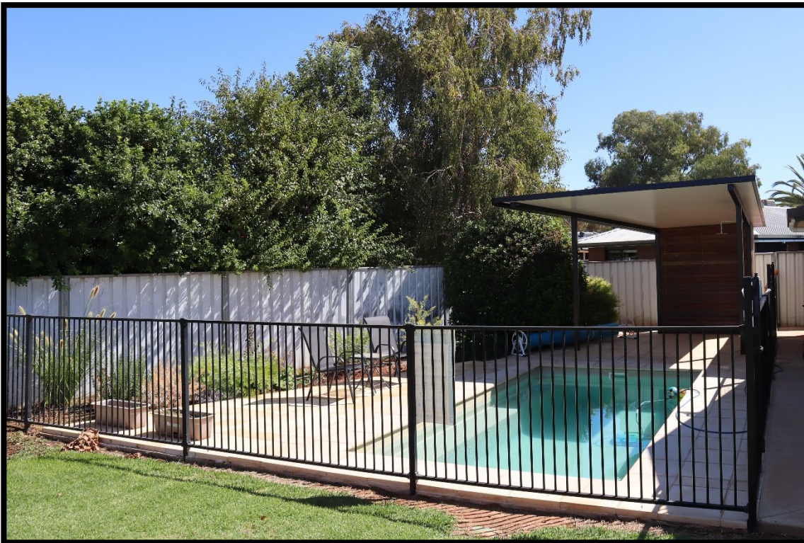
Swimming pool safety barrier, and veranda (located inside the pool safety barrier area)
